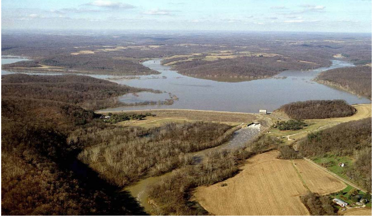
Figure 18. Mohawk Dam, located in central Ohio (USACE photo).
