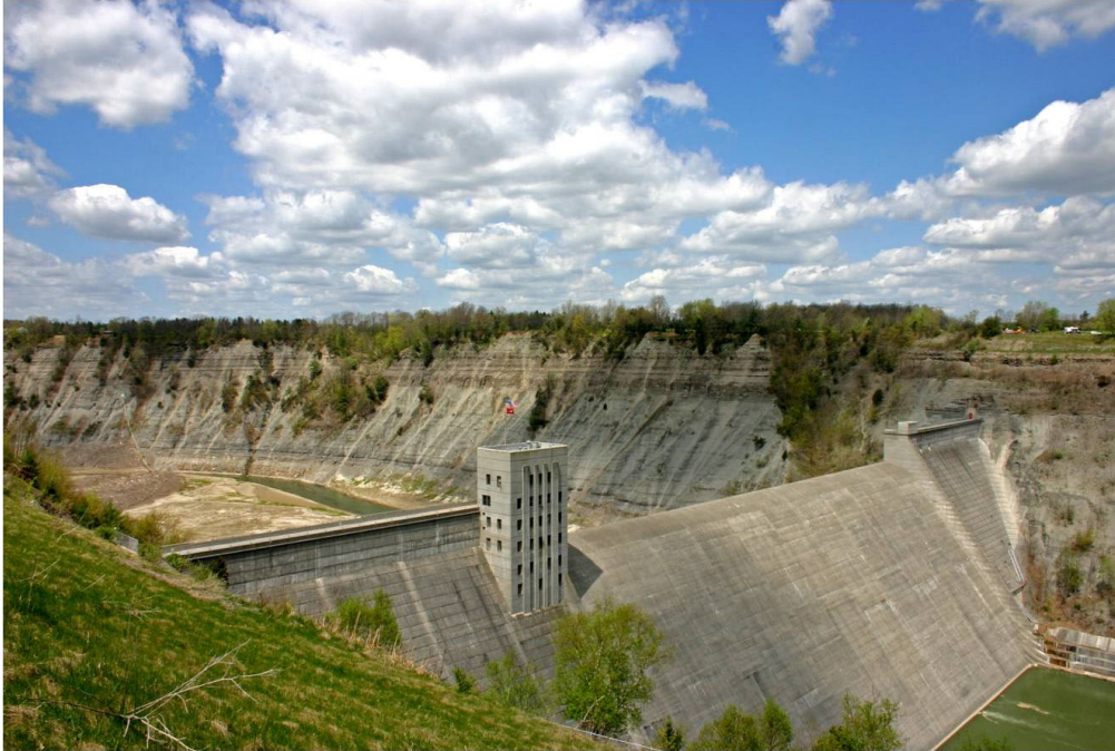
Figure 8. Photo of Mount Morris Dam (photo by Bob Oswald, USACE).
